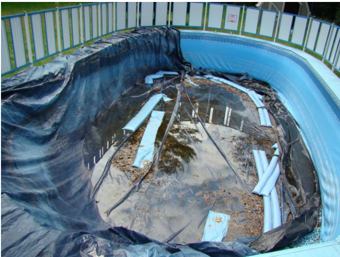
Figure 21. Abandoned swimming pool with collapsed cover collecting water & debris (Topsfield).
