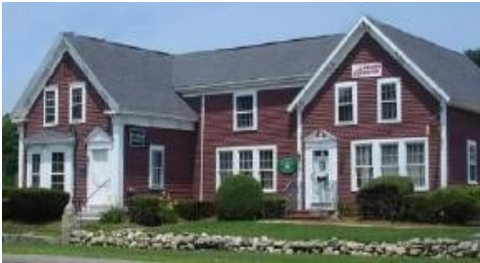
● Figure 3: Example of visual interest while reducing the appearance of bulk with extended gable additions.
