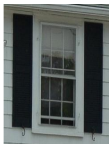
Figure 17: Window with shutters
