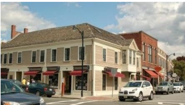
Figure 21: Corner building with attractive entrances and windows facing both streets
