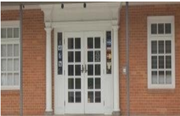
Figure 19: Greek Revival entrance
