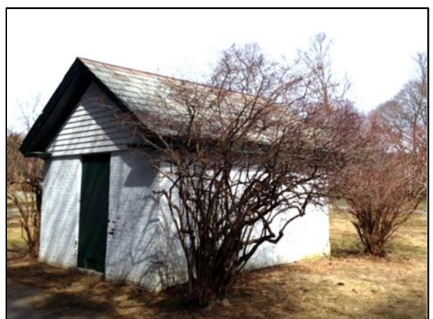
Casket holding house, built in 1877 , was last used about 1970. Photo, J. Hauck, 2018.
