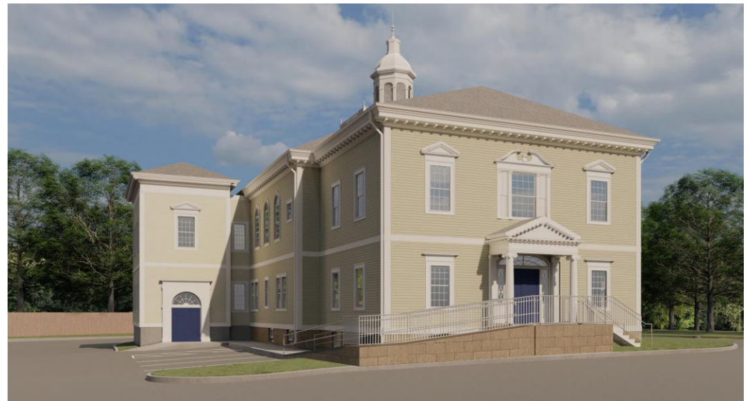
Improvements include an addition to the back of the building to house a new ground level entrance and elevator, as well as a new ADA compliant ramp to the side entrance
