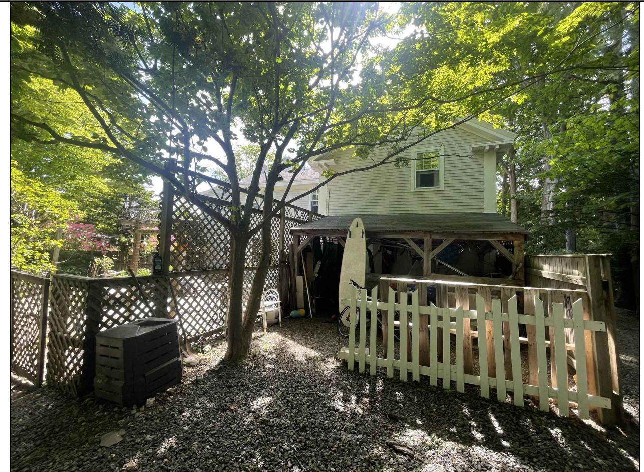
6 REAR ELEVATION OF GARAGE - AREA OF PROPOSED ADDITIONS NOT VISIBLE FROM A PUBLIC WAY
