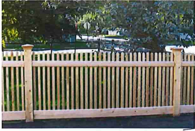
CEDAR PICKET INSTALLED AT POOL CODE HEIGHT
