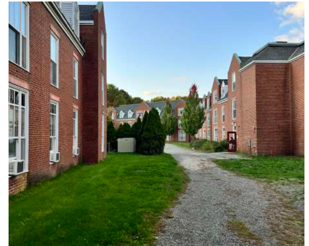
Above: view of the wetland Below: view of Student Housing Buildings E+F
