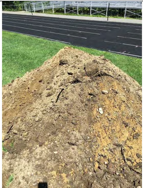
Photo 4: Observed stockpile of material from TP-7.
