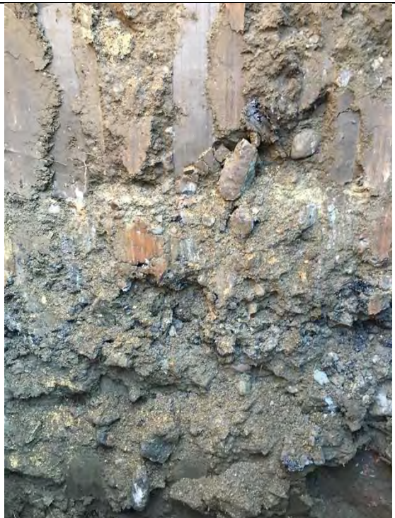
Photo 4: Observed asphalt pavement fill layer.
