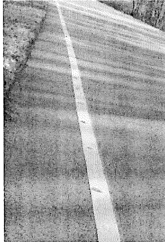
Figure 15: Shoulder. Source: Rumble Strip Implementation Guide
