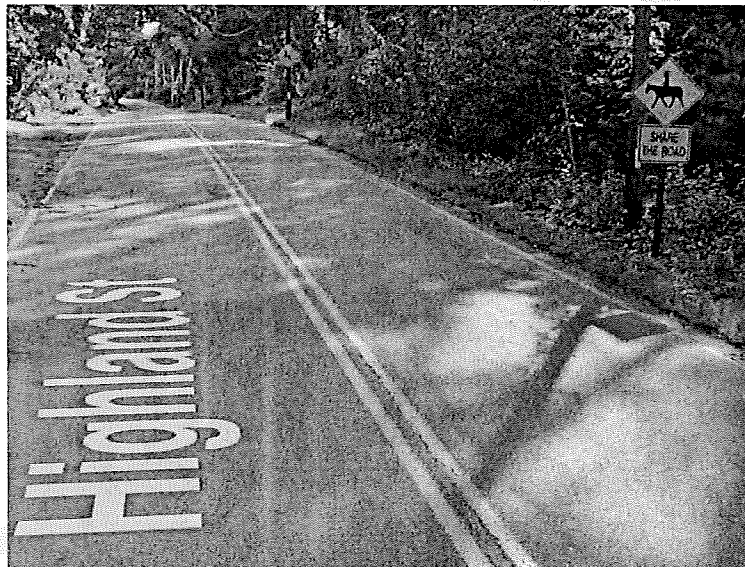
Figure 8: Signages on Highland Street SB. Source: Google Street View (September 2023)
