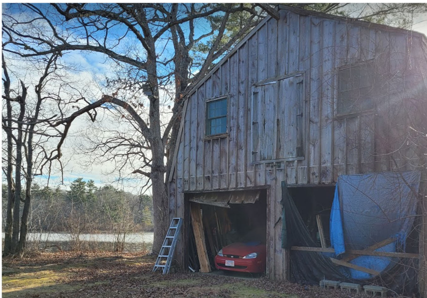
Photo of the existing barn to be renovated within the same footprint. The gravel drive is proposed to be extended to the barn doors for vehicle entry. The gravel driveway is to remain pervious.
