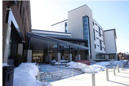
Recently completed portions of the Lowell High School during the ongoing renovation project. JONATHAN WIGGS/GLOBE STAFF/BOSTON GLOBE
